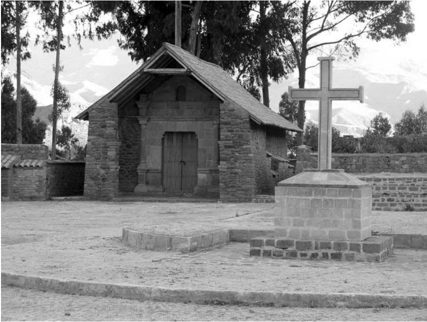
Fig. 9. The chapel of San Sebastian (1565), after restoration.
