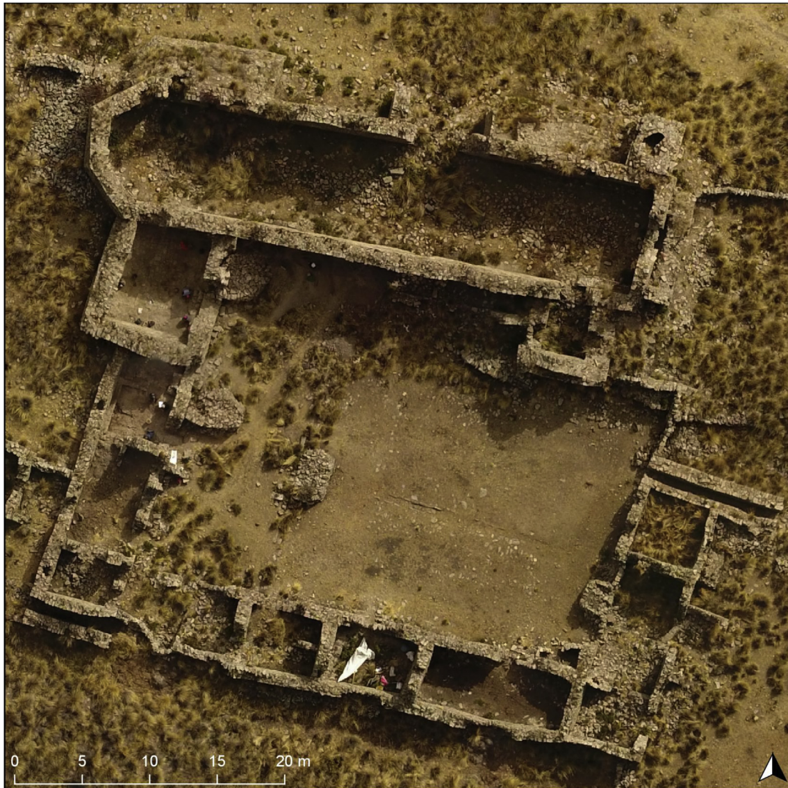
Fig. 6. Example of UAV-based orthomosaic resolution: main church and parish of Mawchu Llacta (with excavations in progress [left]). This 4 cm resolution orthomosaic is derived from 518 photos taken during autonomous UAV survey at a height of 57 m.
